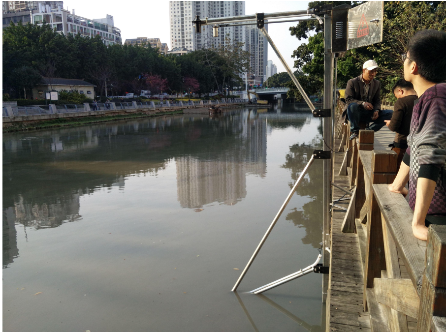
Fig. 31 Installation within River Channel
