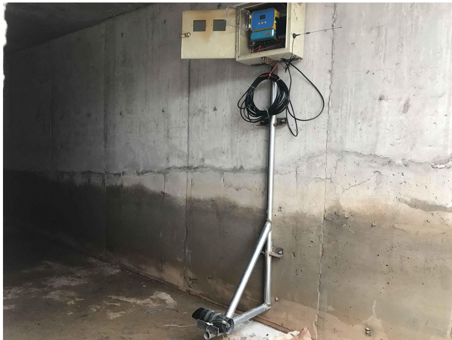
Fig. 30 Installation Diagram within Square Culvert
