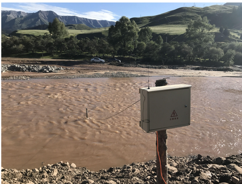
Fig. 19 Completed Installation in Wide River Channel
